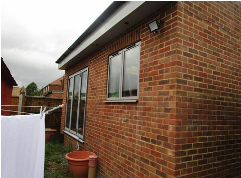
Figure 8: Existing rear extension photograph
